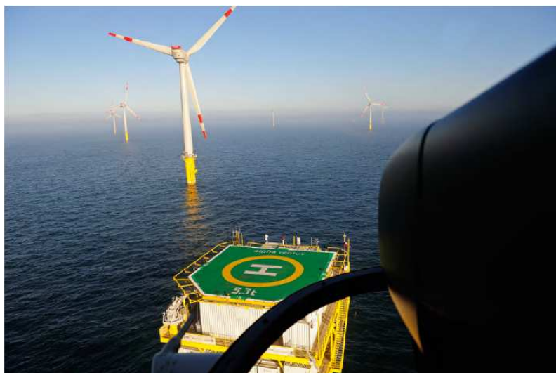
Inspection of offshore wind power plants in the North Sea; Source: Blog Zeit
